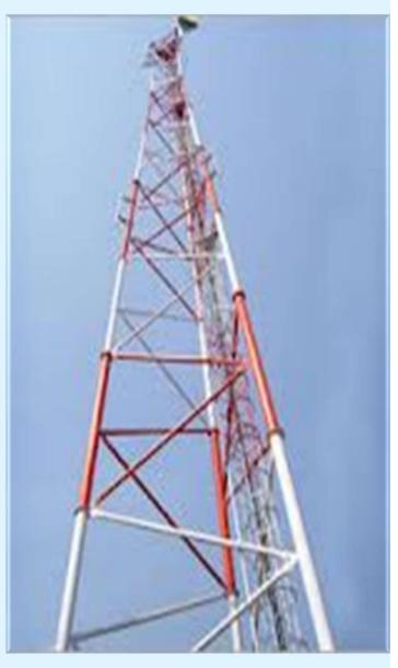
For the urban locations specially narrow base towers are also offered. Final touch is galvanized and if required followed by specific paint.
